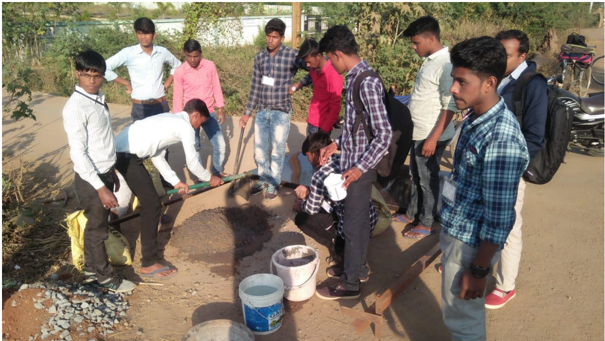
NSS VOLUNTEERS INSTALLING ROAD SIGN BOARDS
